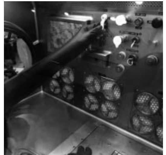
Figure 13. The MSG utility connections.
